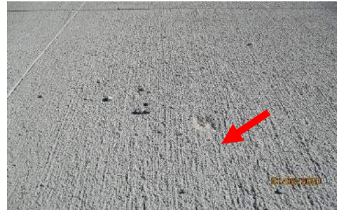
Divots in New Concrete
