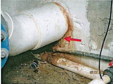
Small Drip Leak near Wall
