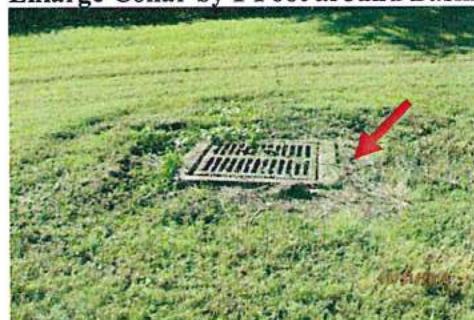
Enlarge Collar by 1 Foot around Basin
