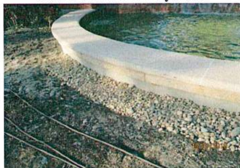
New French Drain System
