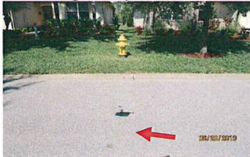
Missing Fire Hydrant Marker
